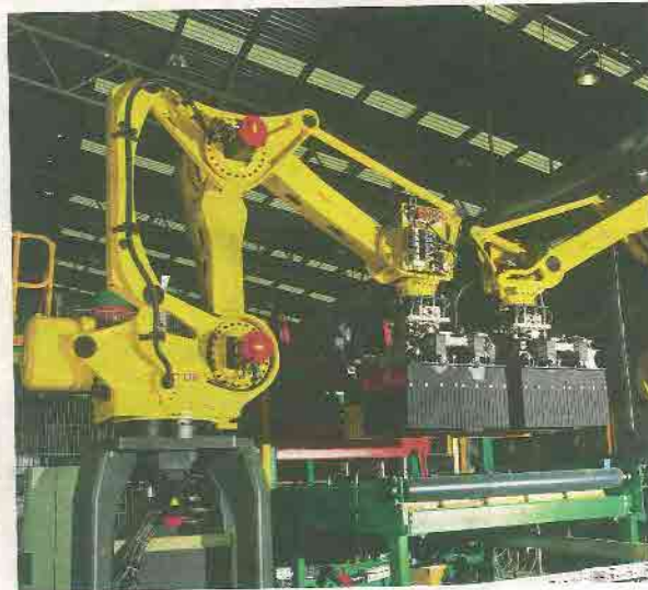
Midland Brick's Kiln number 11. Boral invested over $53 million in 2006 to upgrade production facilities at the Middle Swan brickworks.
